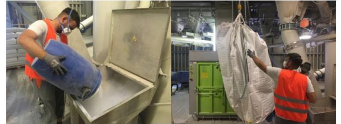
Addition of binders and light-weight aggregates to the plant mix
