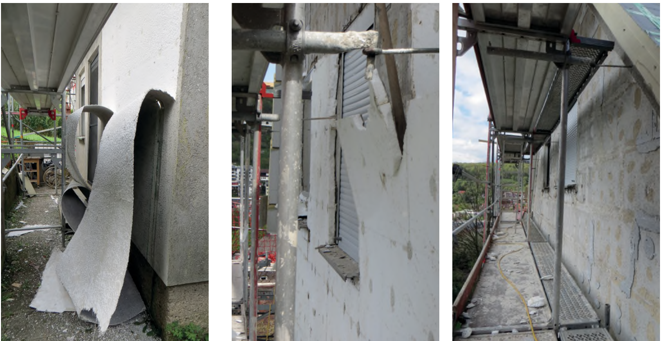
Figure 16 Left: selective dismantling of the rendering system creates a clean insulation surface. Middle: removal of the insulation layer from the wall. Right: stripping of existing ETICS leaves already a relatively clean wall (residuals of adhesive mortar visible). ©Ralf Pasker
